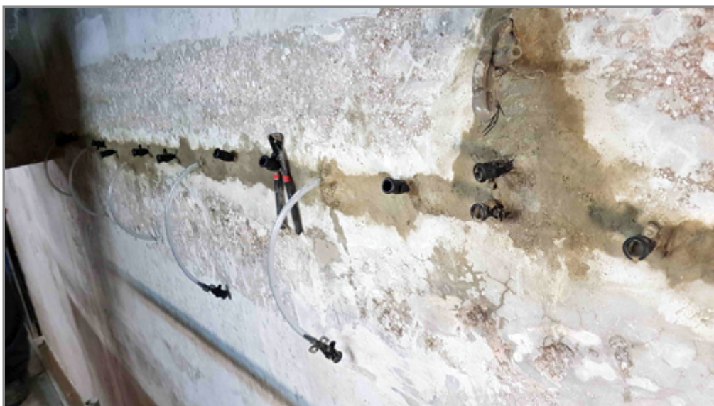
PENETRON INJECT injection points
