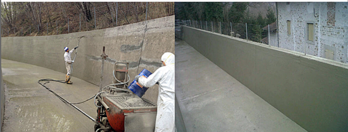
During and after the PENETRON application
