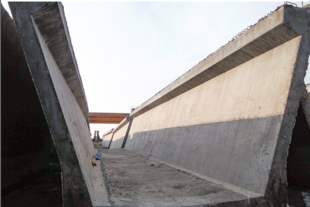
Precast elements at Tidagundi Canal
